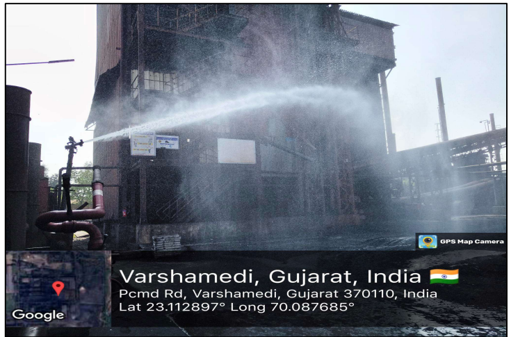
Geo-tagged photographs of water sprinkling facility for dust suppression
