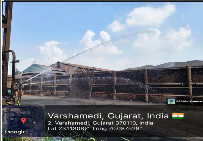
Geo-tagged photographs of water sprinkling facility for dust suppression
