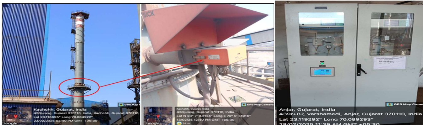
Online CEMS systems installed and real time data uploading to CPCB & GPCB Servers
