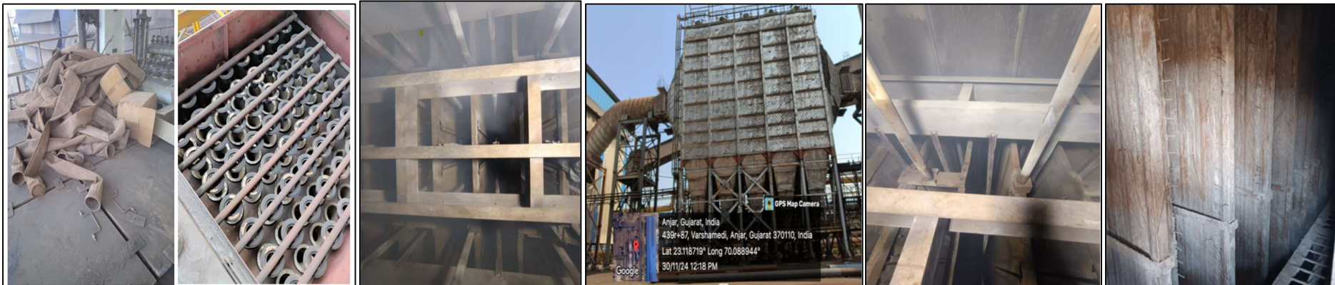
Photographs of the Maintenance of ESP fields & Bags replacement in Air Pollution Control Devices (APCD)
